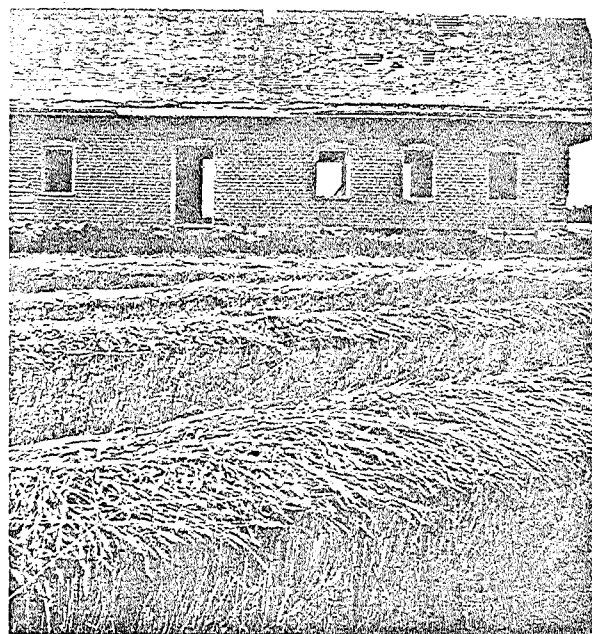
Side view. Note: underlayer of cedar, covered in bricks.
