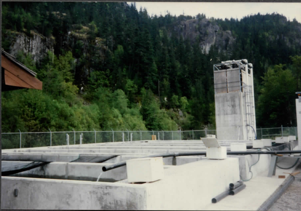
8 concrete raceways with the feeding boxes in the foreground.
