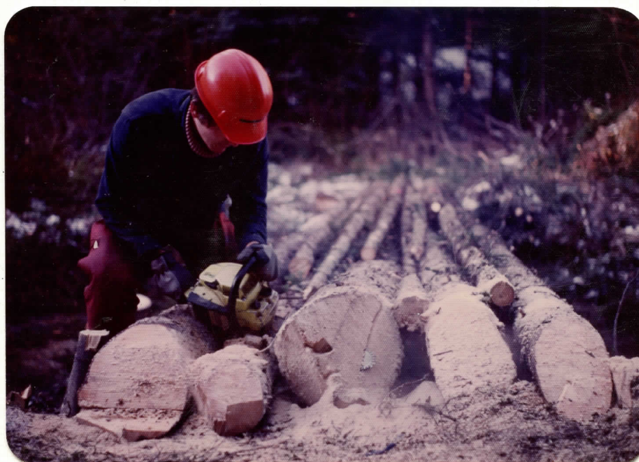
Saw off the end of each log at an angle of approximately 1y 30°. The bridge is completed.
