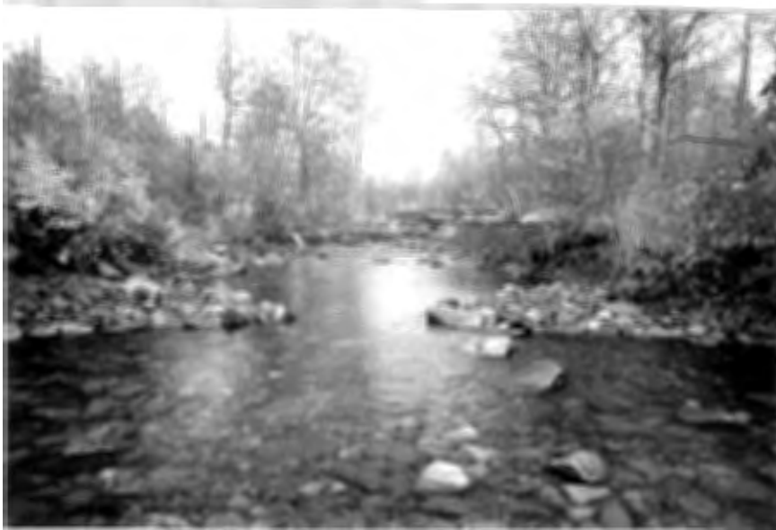
Photo 14 Deflectors in place. Notice large boulders at points of deflectors.
