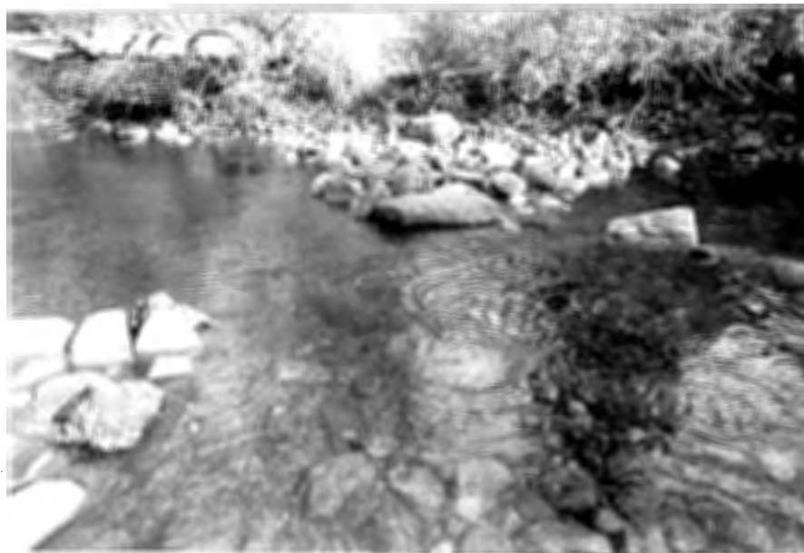
Photo 16 Closer look at deflectors. Notice how water is funnelled between the structures and down the center of the stream.
