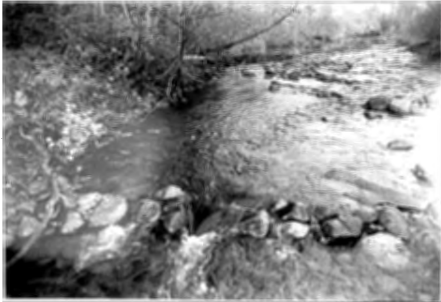
Photo 12 The finished dam. Notice the water being directed into the channel by the deflector, the deflector point is at the upper right in the photo.
